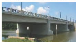
2005-2006, Woody Hayes Bridge Project
