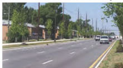
2006-2007, Morse Road Improvement Project
